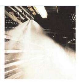
Because water is used in the form of a fine spray, normally no thermal stresses occur that could shorten the life of the protected equipment. This is due to the small droplets creating uniform surface cooling.
