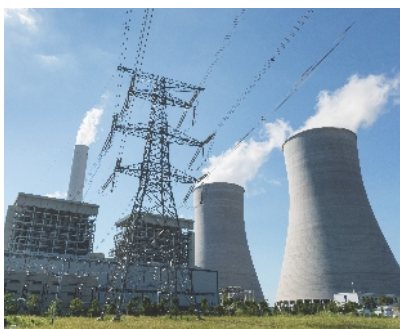
Power generation facilities
