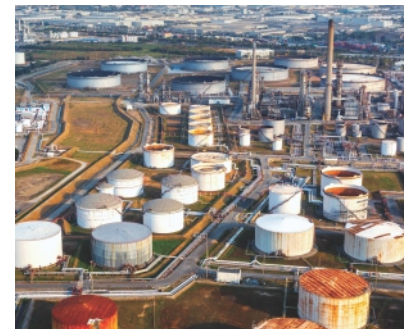
Petroleum and chemical processing plants
