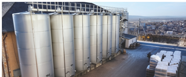
Flammable liquid storage tanks and warehouses
